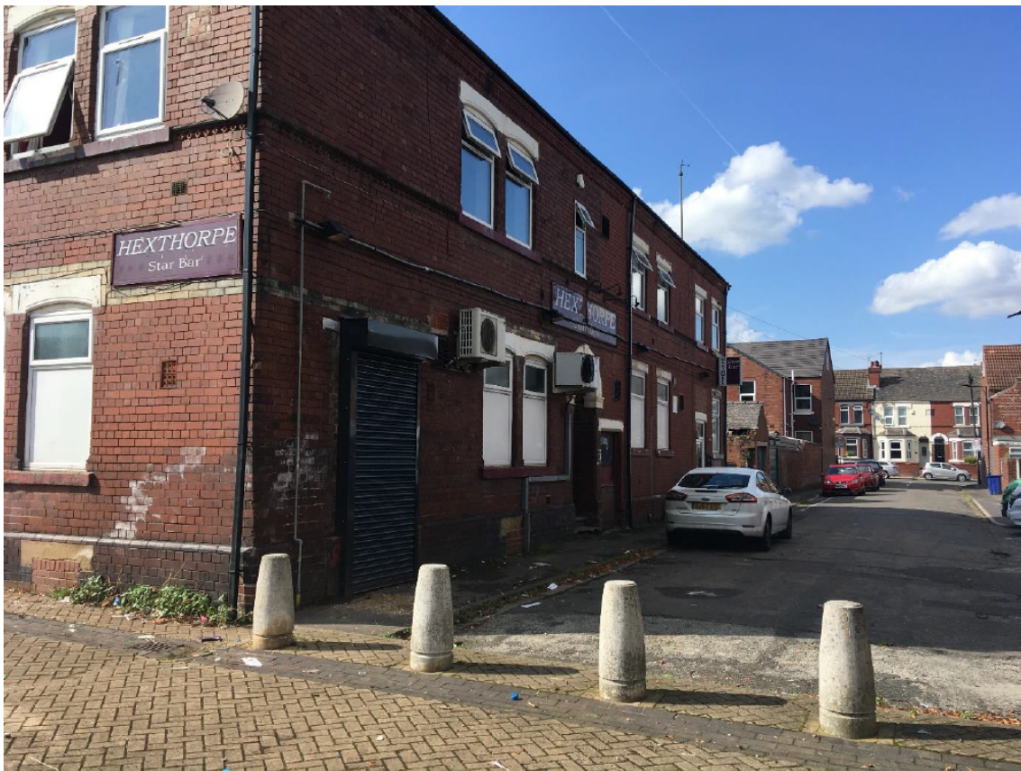
Photo 1: Application Site: Elevation at Langer Street
